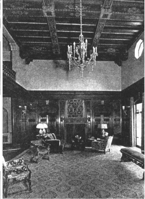
RIGHT: James West's own cabinetmakers in his lumber mills made the walnut paneling for the two-story living room. The Renaissance-style fireplace surround is carved Caen stone. The wood-beamed ceiling features fine ornamental floral and other motifs. Rugs and furnishings, now long gone from the house, included a hand-tufted rug made by Austrian weavers and Ferez sofas and chairs covered in brocade and cut velvet.
